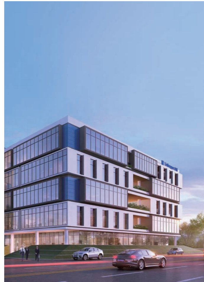
Unihopper R & D Building 库博研发大楼
